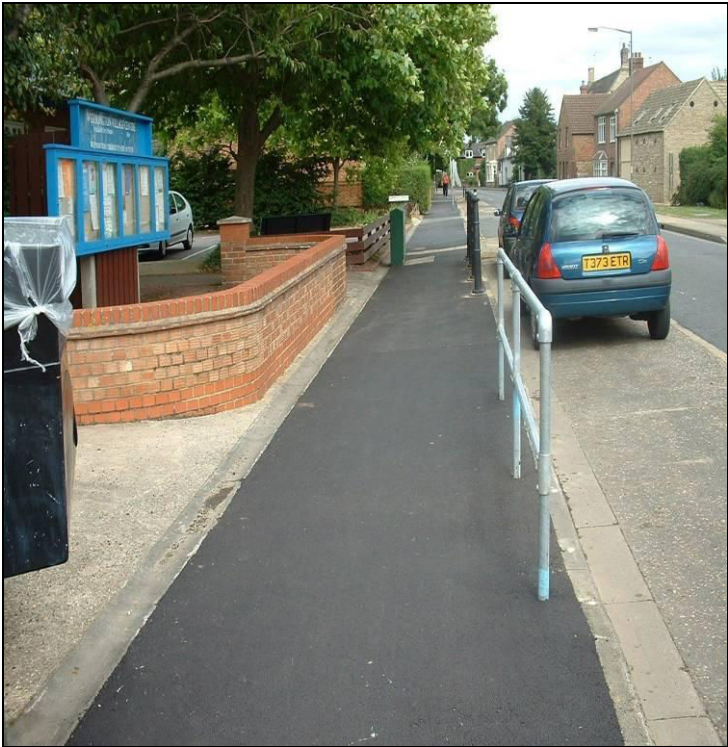
Figure 10 Footway in Church Street, Werrington after Slab Replacement
