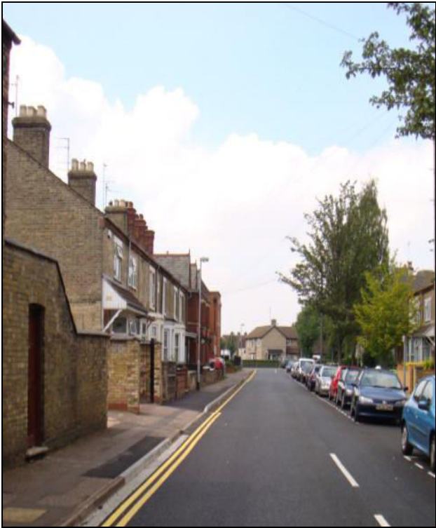
Figure 8 Manor Street after Resurfacing, kerb and drainage improvements
