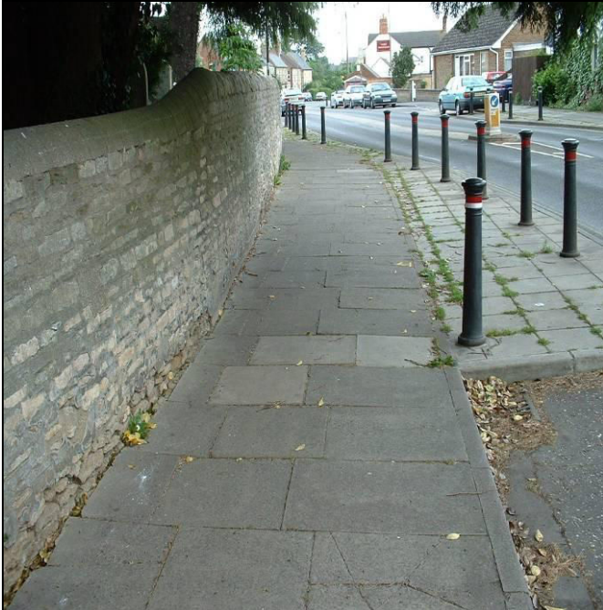
Figure 6 Footway in Church Street, Werrington before Maintenance
