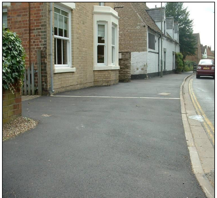
Figure 18 Church Street Werrington after Slab Replacement Scheme
