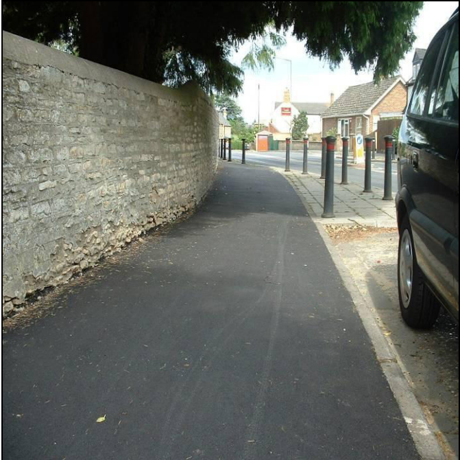
Figure 7 Footway in Church Street, Werrington after Maintenance
