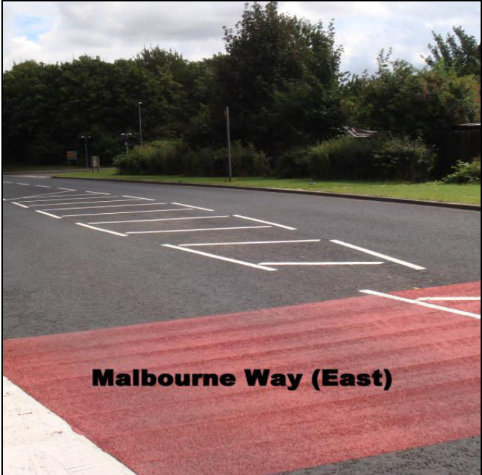
Figure 5 Malbourne Way after Resurfacing
