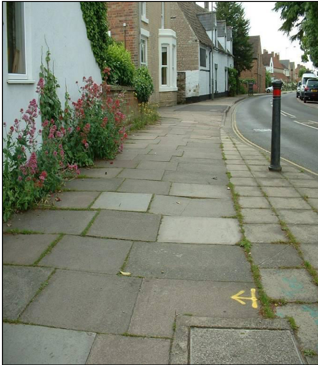
Figure 17 Church Street Werrington before Slab Replacement Scheme
